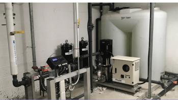
Onsite Water Reuse Systems (OWRS) will be required to collect AC condensation and rainwater, and are allowed to be used for irrigation, toilet flushing, and cooling towers. To help facilitate the implementation of OWRS, Austin Water offers several incentives as part of its Go Purple Program.
