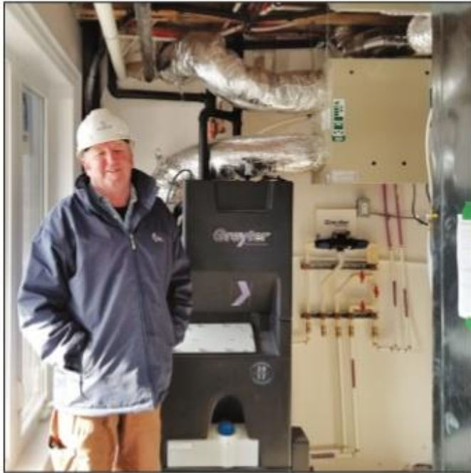
Jim Couperthwaite of Geranium Homes with newly installed Greytex HOME system. Upper right: Typical Model slab on grade design due to high water table. Right: Two-stage furnace with tankless hot water heater for radiant floor and domestic hot water.
