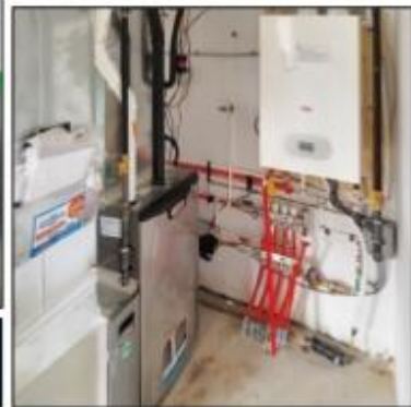
Jim Couperthwaite of Geranium Homes with newly installed Greytex HOME system. Upper right: Typical Model slab on grade design due to high water table. Right: Two-stage furnace with tankless hot water heater for radiant floor and domestic hot water.
